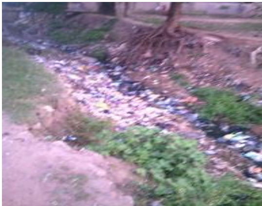
Fig. 2b: Lateral expansion of the gully due to mass wasting
