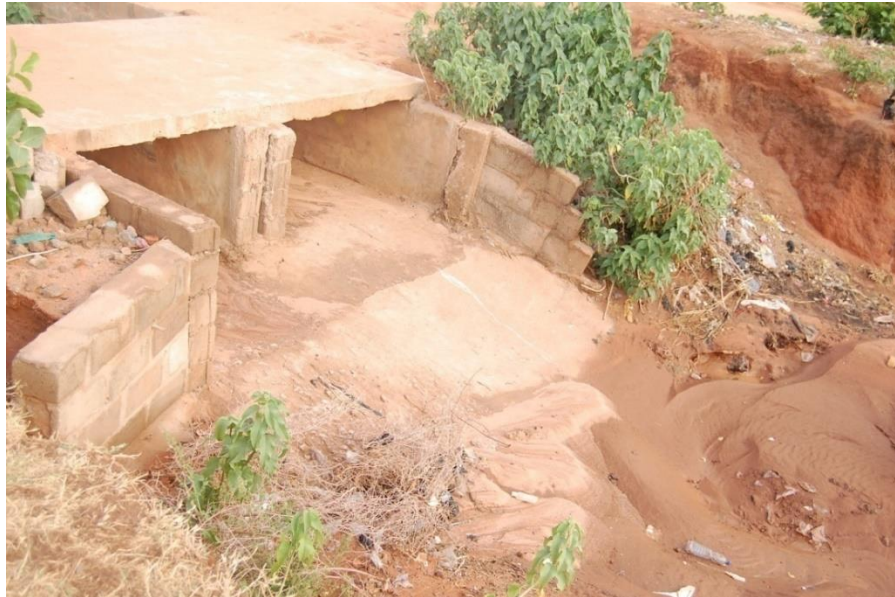
Plate 2: Collapsed Culvert along the gully site
