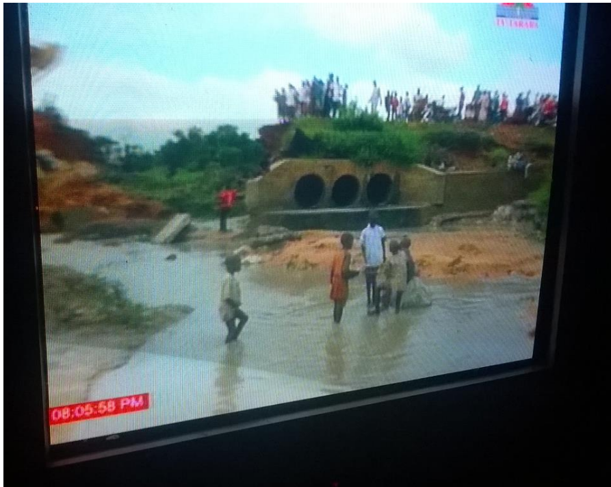
Plate 2: Bridge collapse at Maraban Gassol in Taraba State
